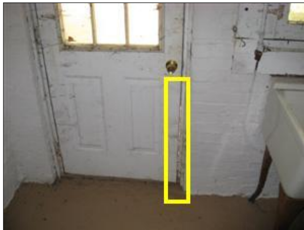
2.1 Picture 1 Basement entry
