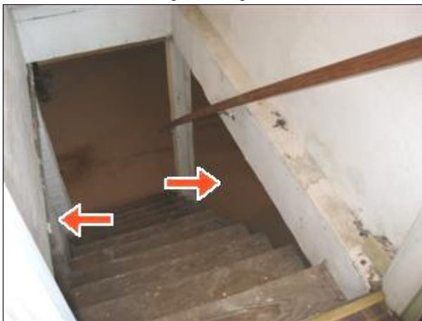
3.3 Picture 1 basement stairs
