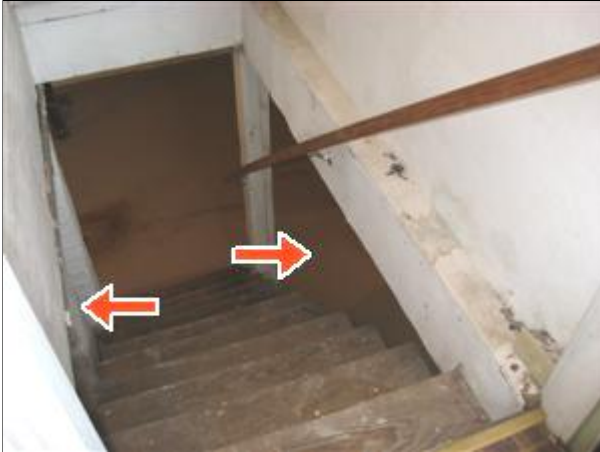
3.3 Picture 1 basement stairs
