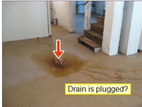
5.0 Picture 4 basement floor drain
