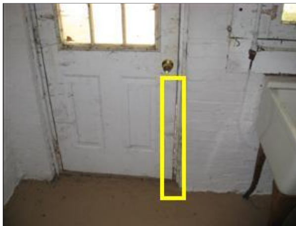
2.1 Picture 1 Basement entry
