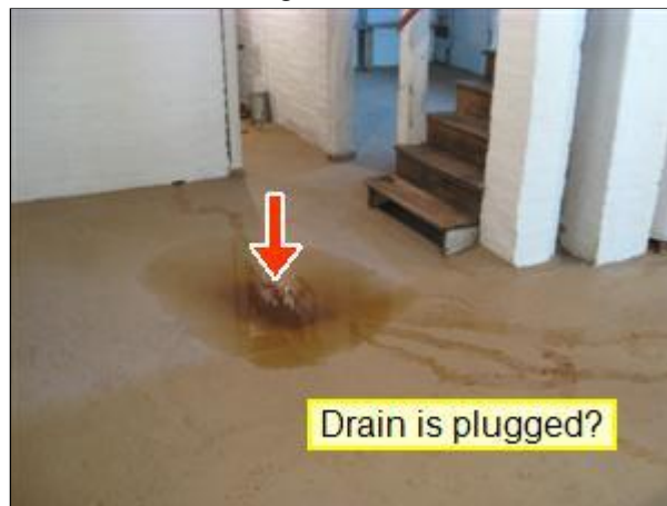
5.0 Picture 4 basement floor drain
