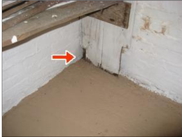
4.0 Picture 2 basement wall
