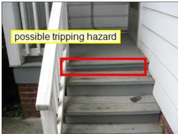
2.3 Picture 2 Rear Porch
