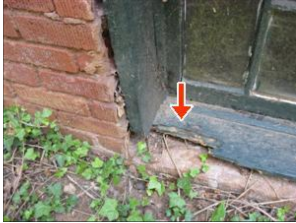
2.2 Picture 1 Basement window (s)
