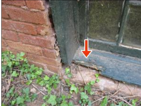
2.2 Picture 1 Basement window (s)
