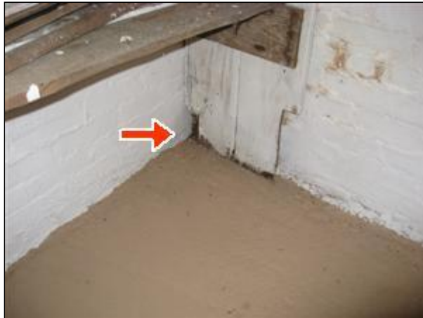
4.0 Picture 2 basement wall
